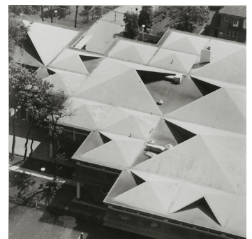
Roof of the Shell canteen [1976] featuring triangular, pyramid-shaped roofstructure.
