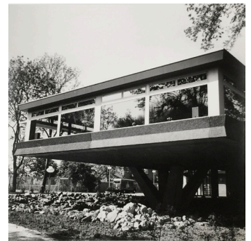
Shell canteen [1976] featuring concrete columns and gravel concrete floor belts.
