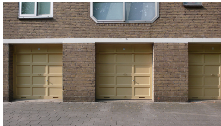
Detail of ground level showing the refined detailing of the garage boxes in 2020.
