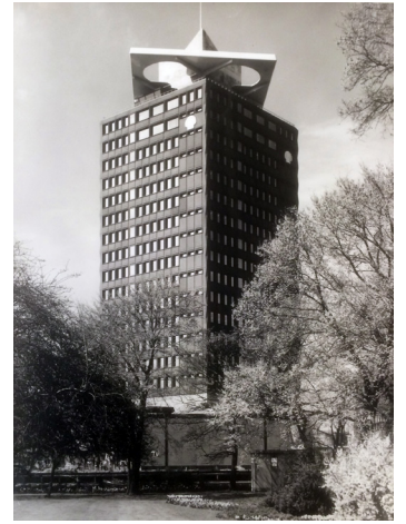
43. The Shell tower in Amsterdam North.
