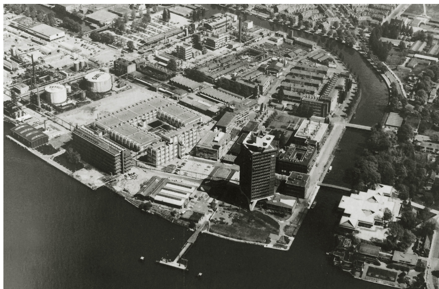
The Shell technology campus with the Shell tower in front and the Shell canteen on right the North Banks of the IJ river [1976]. Image: Sandra Guarda "The Importance of Being Overhoeks"
