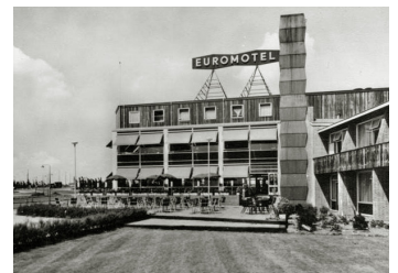
14. Euromotel Joan Muyskensweg [1962]. Upon completion, this Euromotel was the largest motel in Europe. (Demolished)
