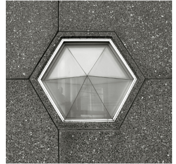
27. Hexagon window in the gravel concrete ground level underneath the Shell tower in 2012.
