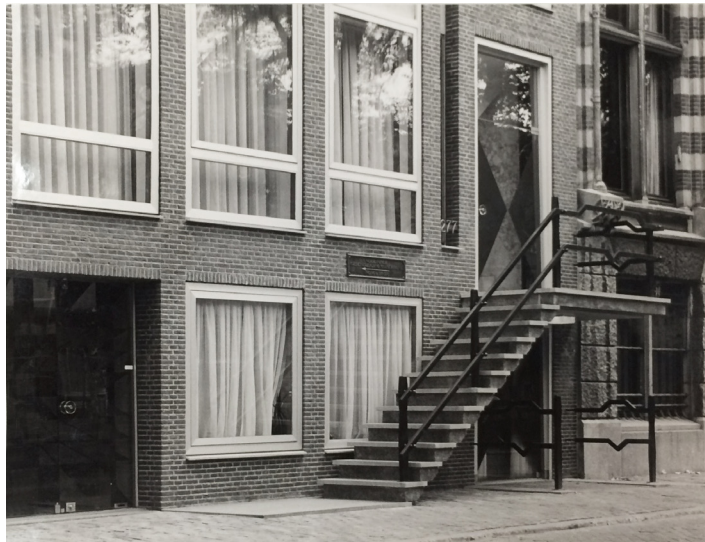
42. Main entrance stair to the piano nobile with original glass front door and subtle house number 277.
