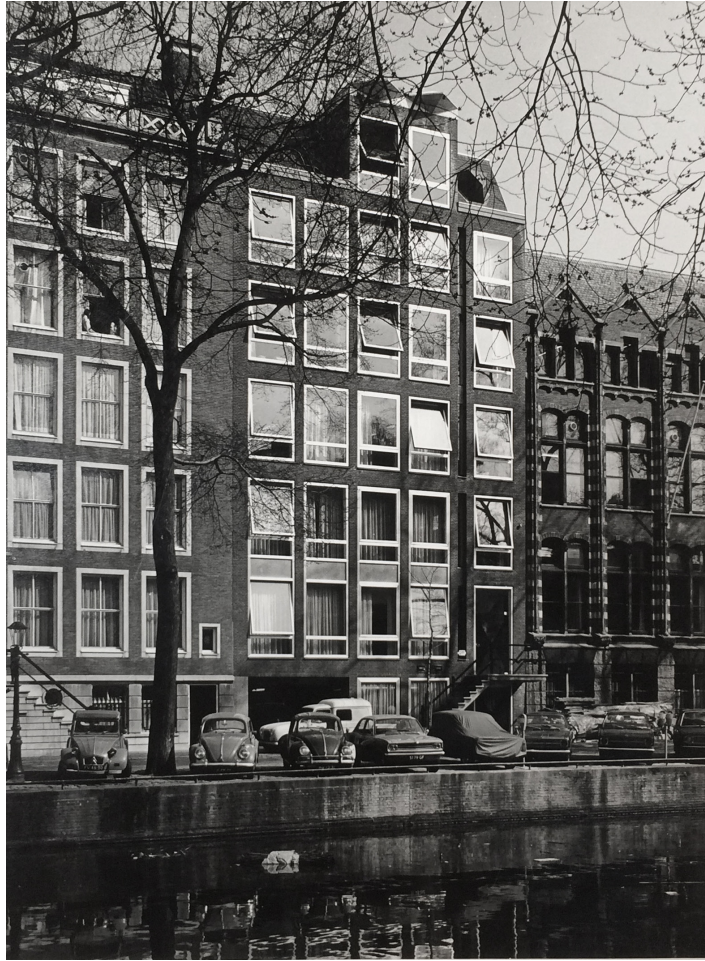
Office building in between canal houses on Keizersgracht [1968], with the pivot windows that gives the facade an very dynamic appearance.
