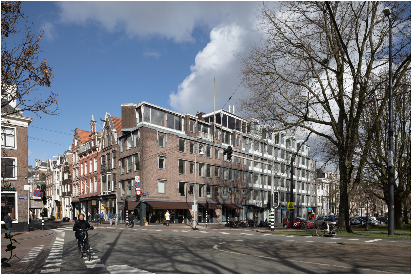
The office building with shops on ground level at the end of the Utrechtsestraat. Image: Bart van Hoek [2020]
