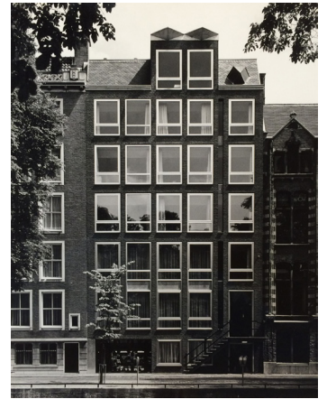
41. Office building at Keizersgracht 277 [1968].
