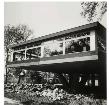
Shell canteen [1976] featuring cantilevered concrete pylon and gravel concrete floor belts.
