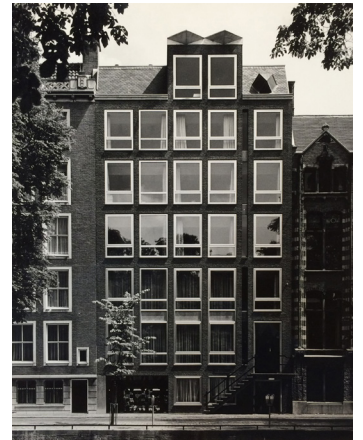
41. Office building at Keizersgracht 277 [1968].
