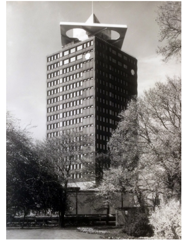
43. The Shell tower in Amsterdam North.
