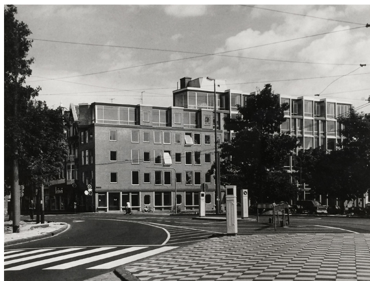
The elevation facing the Frederiksplein in the late 1960s, with some opened pivot windows.
