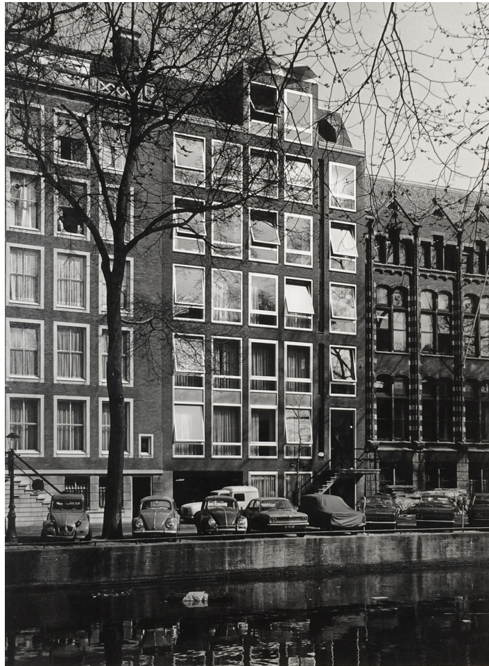
Office building in between canal houses on Keizersgracht [1968], with the pivot windows that gives the facade an very dynamic appearance.
