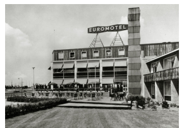
14. Euromotel Joan Muyskensweg [1962]. Upon completion, this Euromotel was the largest motel in Europe. (Demolished)
