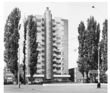
2. The Skyscraper [1932], the first high rise building in Amsterdam by J.F. Staal.
