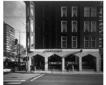
22. Former bank branche on the corner Stadhouderskade/Van Woustraat with characteristic natural stone interventions on the ground floor [1974].
