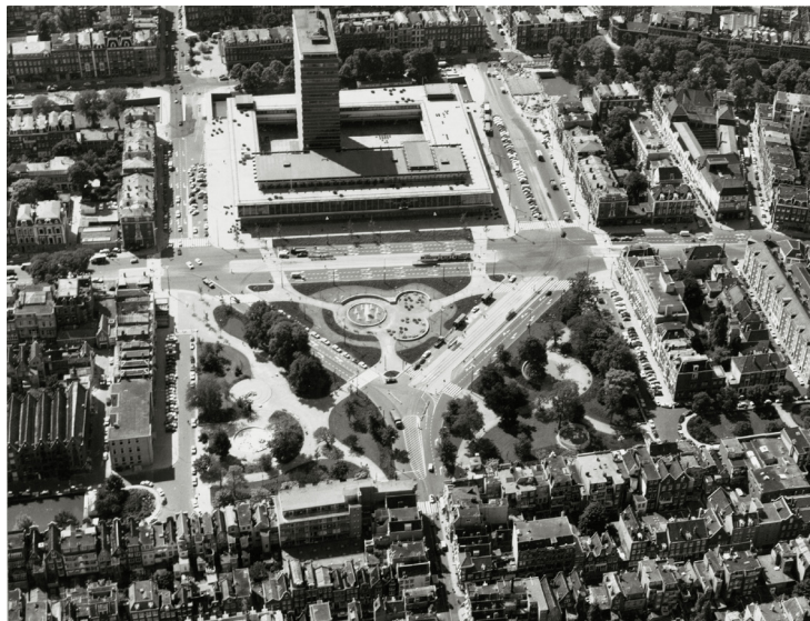
Fredriksplein with the office building at the bottom and De Nederlandsche Bank in the top in de late 1960s.
