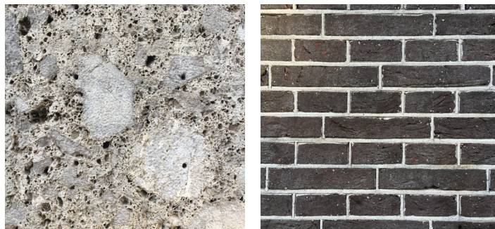
Typical coarse natural stone and brickwork in cross bond in project on Haarlemmerplein [2020].
